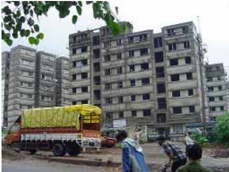
Figure 5. Photograph of JVLR resettlement construction site, July 2004.
